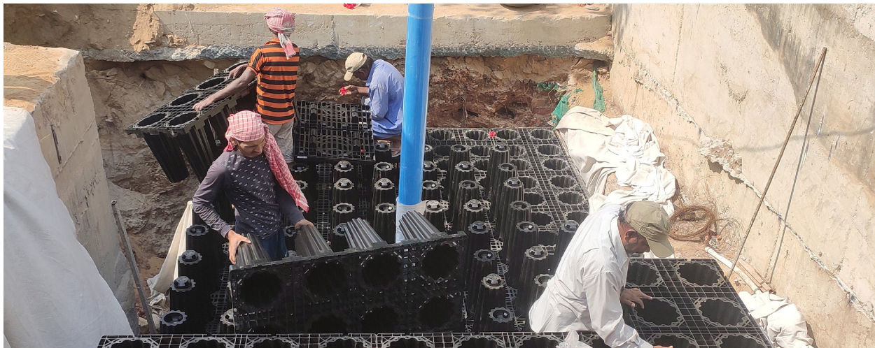
Installation of ACO StormBrixx SD 900 modules in progress – designed for efficient assembly
