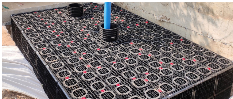
Installation of ACO StormBrixx SD 900 modules in progress – designed for efficient assembly
