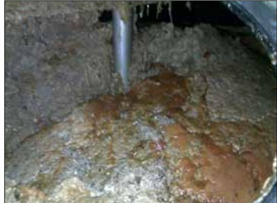
Heavy accumulation of fats, oils, grease and sludge in a grease separator due to missing regular disposal of contents.
